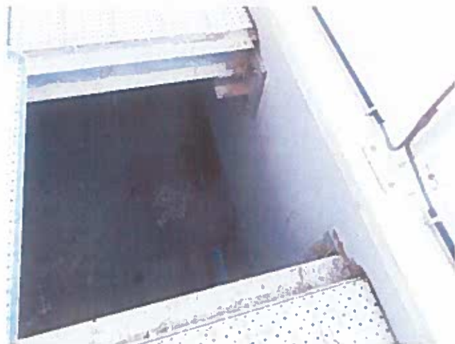
Oil Filled Step Up Transformer Bund wall below gratings
